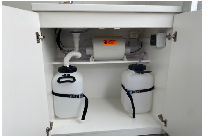
Heisswasserboiler, 2 Wassertanks
